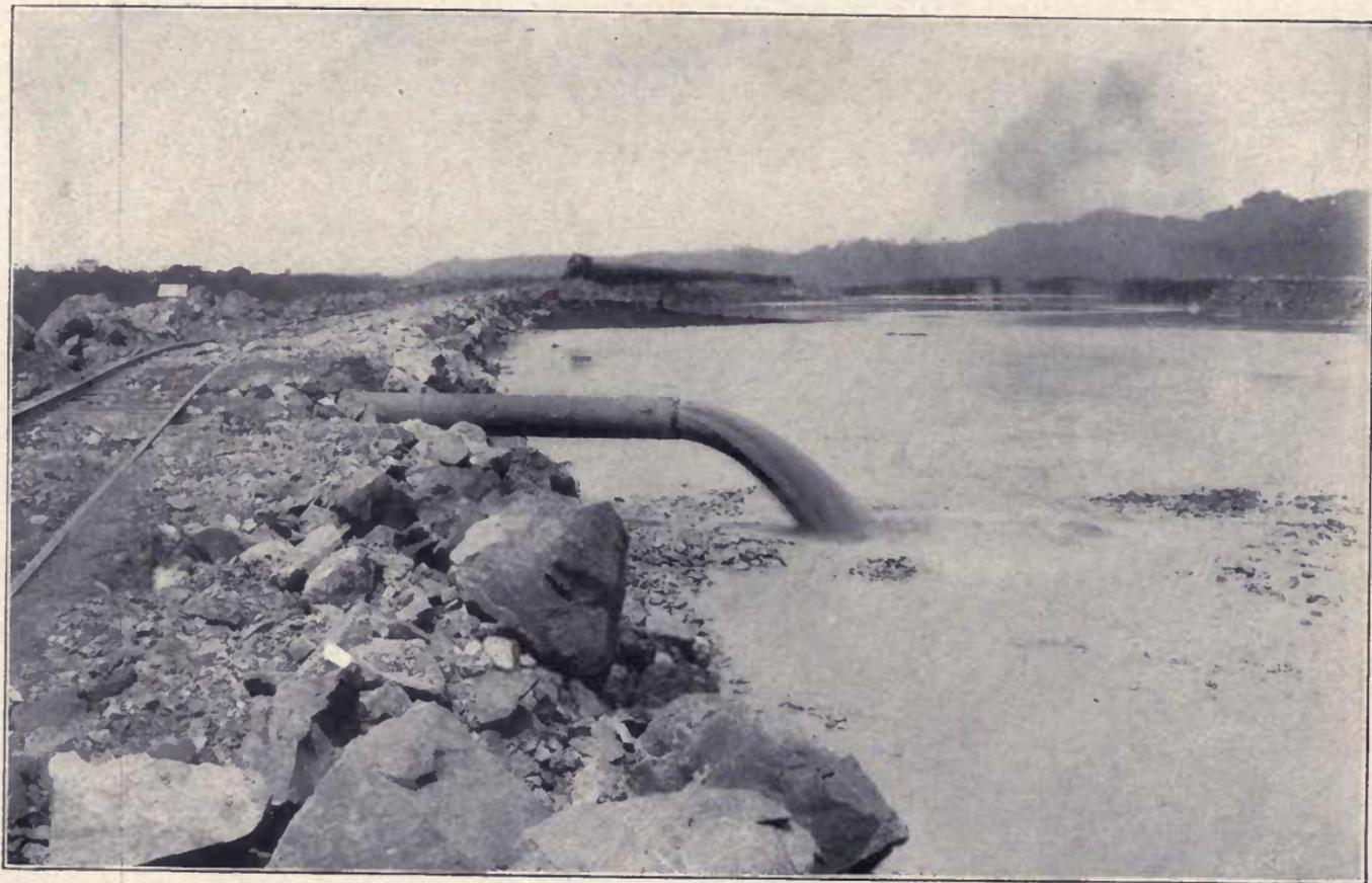
Gatun Dam, East Section, Showing Discharge from Suction Dredge, with Hydraulic Fill, Looking West
